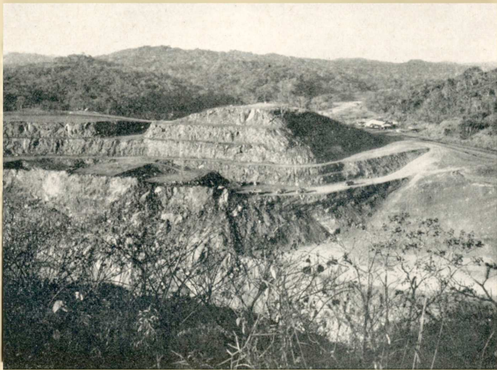
CONTRACTORS HILL, less than a year ago a towering mass of rock and earth, is now a series of great terraces. From Gold Hill, on the opposite side of narrow Gaillard Cut, the hill looks like a staircase for Paul Bunyan.
