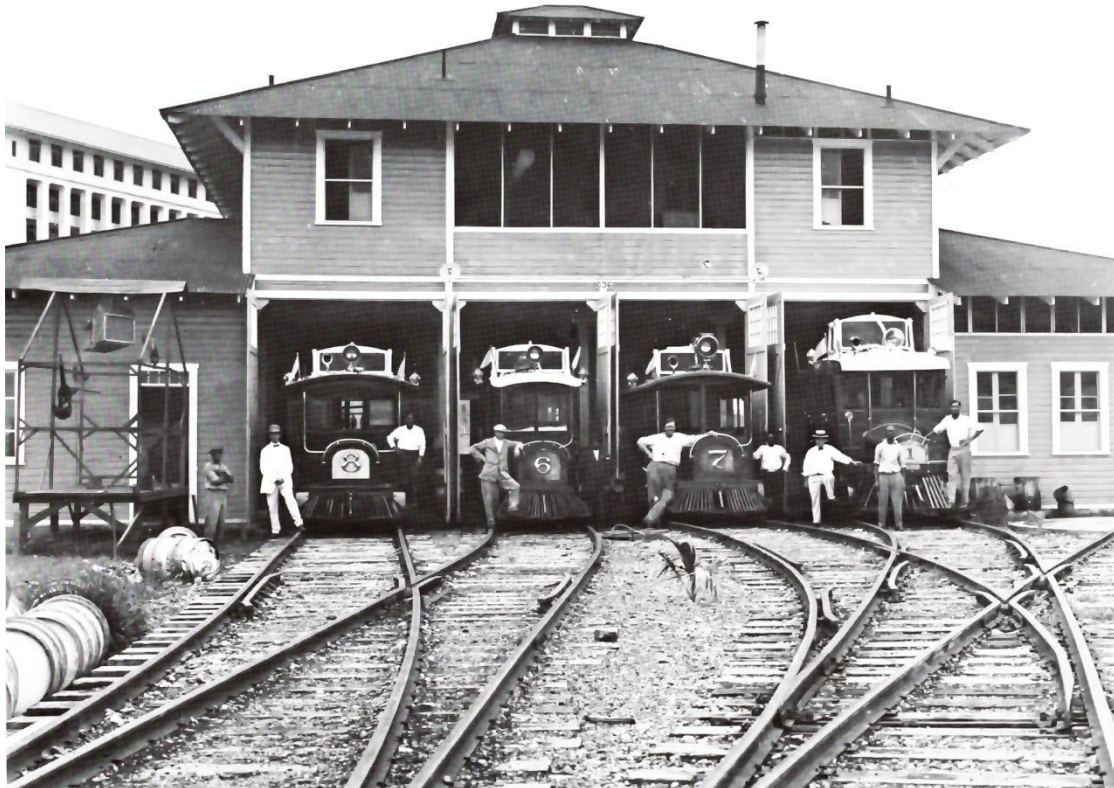
Fig. 2. When the new administrative building was built at Balboa Heights a home for the motor cars was built at Balboa. Because they were called motor cars their home was called a garage. It was located just west of the Balboa Heights station. The motormen were known as chauffers. PCC 1574
