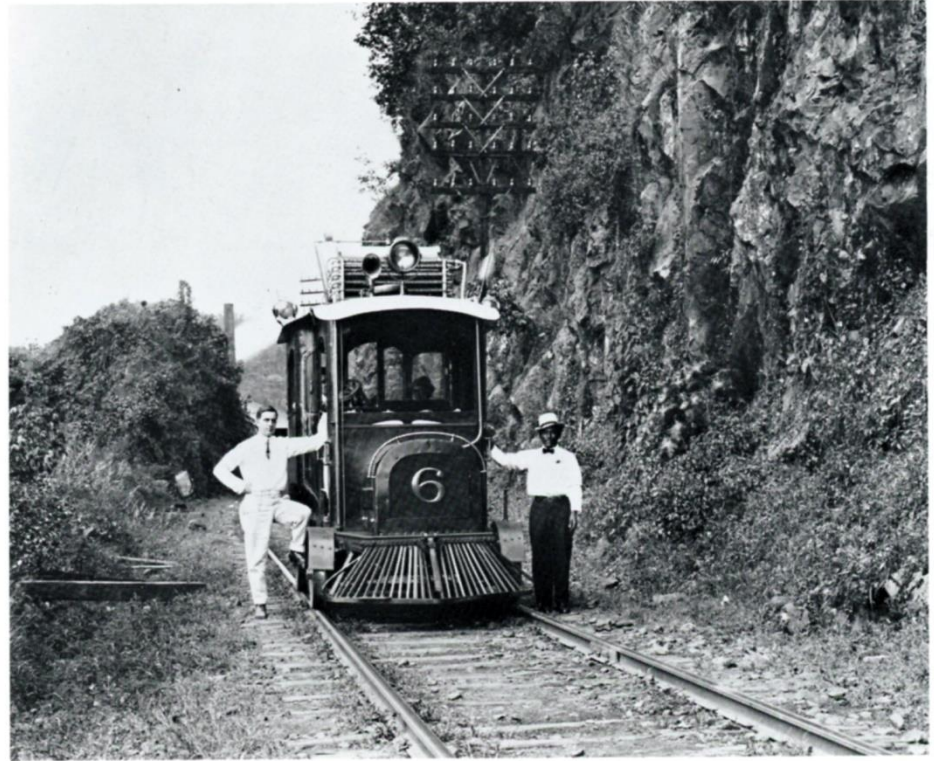
Motor car No. 6 is at the summit of the 1907 diversion of the original P.R.R. behind Contractor's Hill during 1911. PCC 1539
